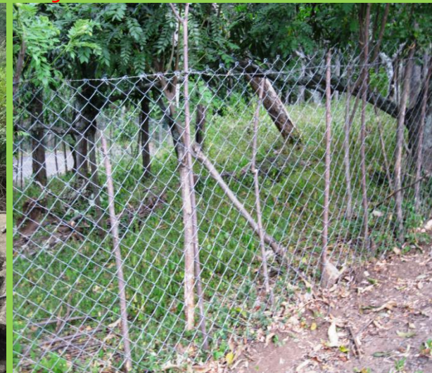
Integrated barbed wire and life fencing which is safe for animal and protection for agricultural cultivation.
